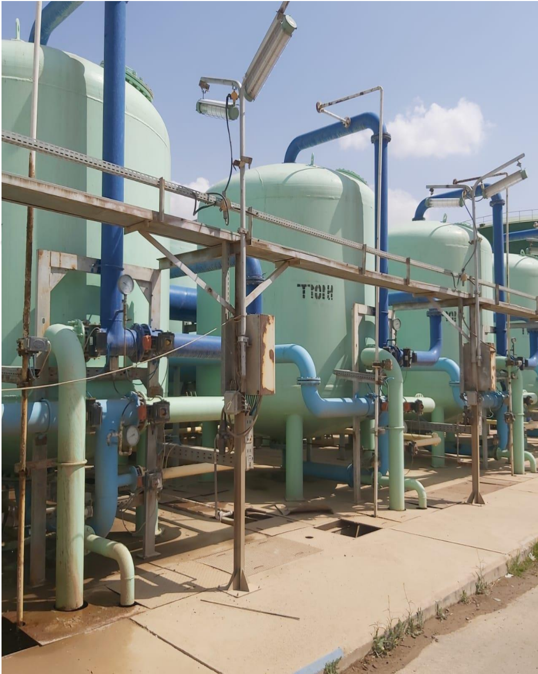
Figure (3.11) Model of a Backwash System of sand Filters Specific to the Specifications of the Tigris River water.
