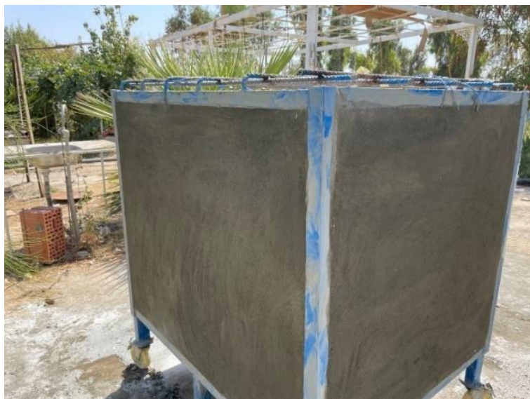
Figure 3.5. The exterior walls are covered with Cement plastering
