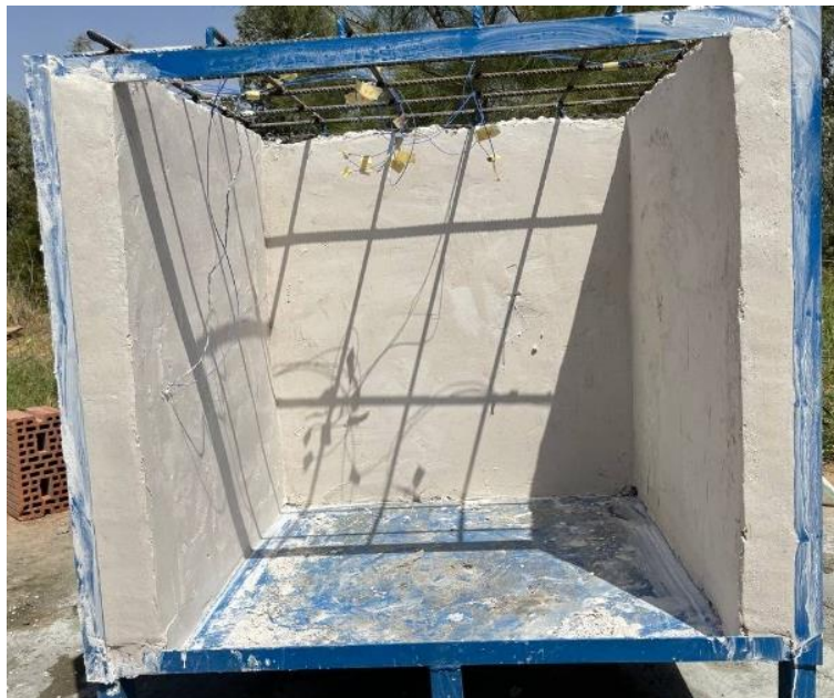
Figure 3.3. The inside walls are covered with Gypsum plastering.
